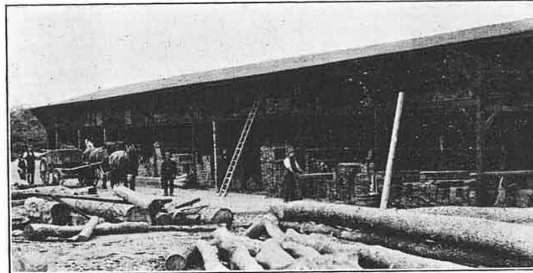
TIMBER SHEDS—WESTERHAM YARD.
