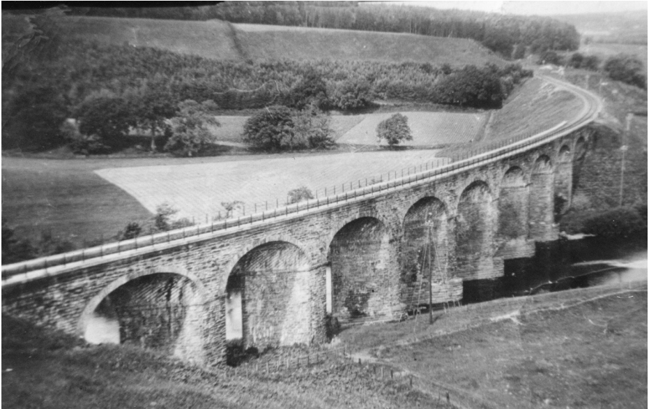
Looking over Riddings Viaduct towards Langholm.
